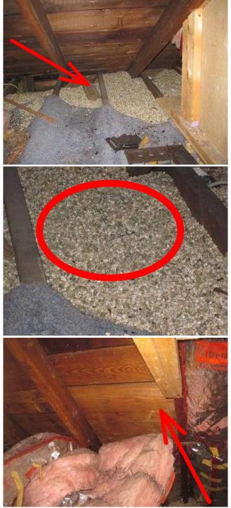
Marginal Not Present Not Present Insulation Depth: 6" Insufficient insulation present Vapor Barrier: Attic Fan:
