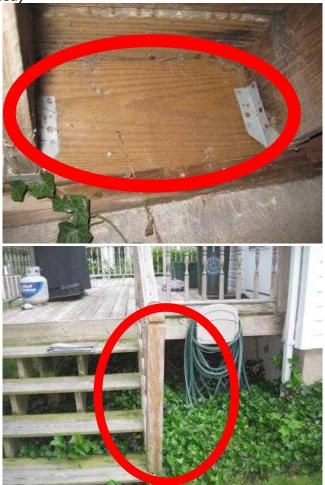
AcceptableGrading: Minor slopeNot PresentSwale:MarginalVegetation: Ivy, Vines Ivy/vines growing on structure,removal is suggested.Not PresentWindow Wells:Not PresentExterior Surface Drain:Not InspectedFences:
