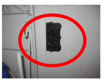
DefectiveElectrical: 110 VAC outlets and lighting circuits Non-GFCI circuit -recommend GFCI circuit be<br/>installedAcceptableCounter/Cabinet: Composite and woodAcceptableSink/Basin: One piece sink/counter top
