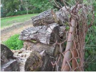
AcceptableGarage Doors: Insulated aluminumAcceptableDoor Operation: ManualAcceptableExterior Surface: Vinyl siding Wood siding in contact with soil. Promotes termites.
