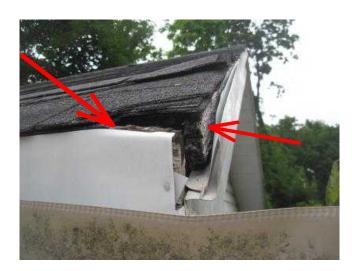
Marginal Acceptable Defective Roof Structure: 2x6 Rafter Trim boards rotted. Ceiling: Exposed framing Walls: Exposed framing Termite damage
